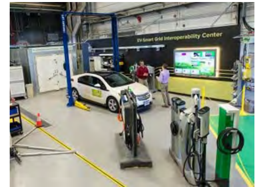
Smart Energy Plazas at bldgs 300 and 362
